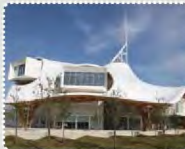
Centre Pompidou Metz
